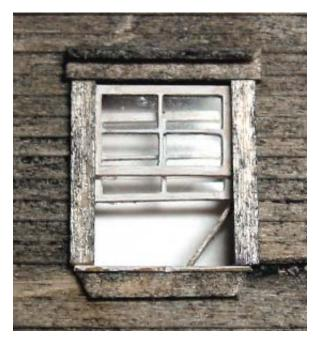
The above finished window shows a double sash with a stick proping the lower sash open. Also note the addition of a second piece of trim across the top of the window as a drip cap. This piece is laid almost flat, slight angle so water would run off.
