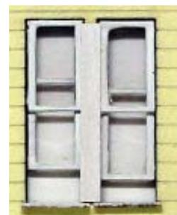
***Photo at right shows both the back and front of a single sash window and a double sash window install. The lower sash in the double sash window has been installed at the half open position which adds some extra character to the building.***
