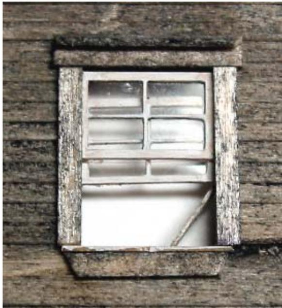
***The above finished window shows a double sash with a stick propping the lower sash open. Also note the addition of a second piece of trim across the top of the window as a drip cap. This piece is laid almost flat, slight angle so water would run off.***
